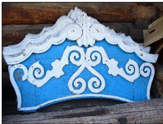
Fig. 1. Window frame upper part (ochélie) from the village of Nizhny Zhirm. Museum of Old Believers' Culture in Tarbagatai village
